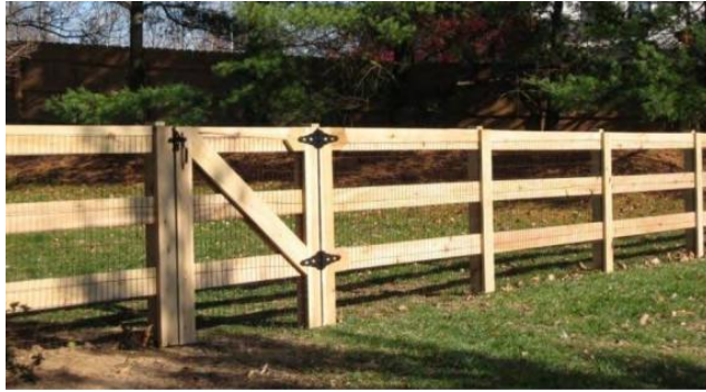
Figure 1108-D: Example of where wire fencing has been mounted on the interior of an approved three-rail fence.
