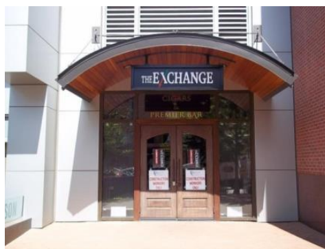
Figure 1116-D: Example of a canopy and related sign
