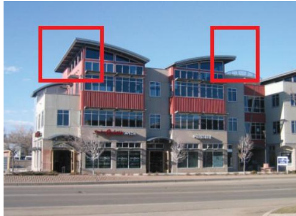
Figure 1109-D: Example the use of eaves, highlighted in red rectangles.
